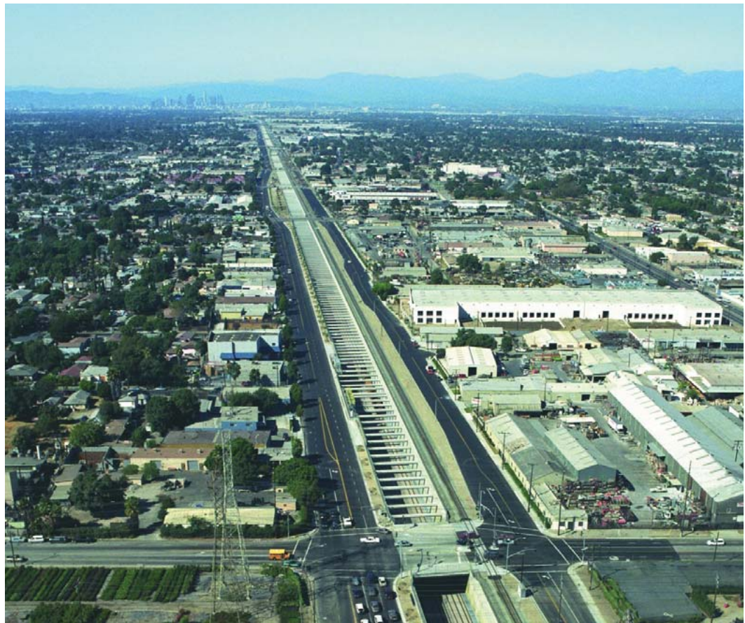
The Alameda Corridor Project built a rail access network to the ports of Long Beach and Los Angeles.
